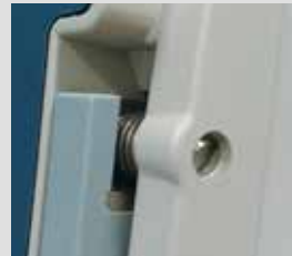
Figure 3: Properly installed (recessed) pivot latch screw
